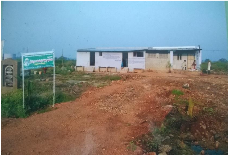
Old Building of the Foundation
